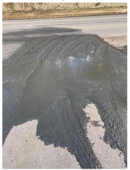
April 2023 Raw sewage seeping out of manhole and spreading down driveway on Church Street
