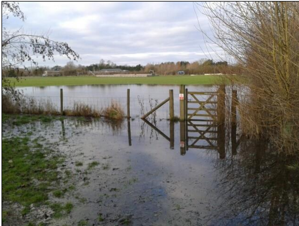
Figure 5. Flooding of the recreation ground in February 2014, viewed from the northern boundary of the development site.
