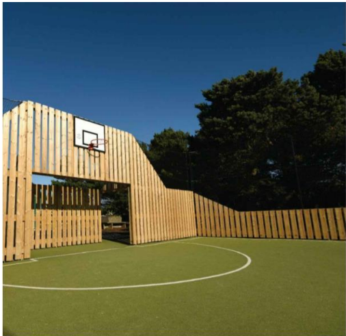
Timber fencing to MUGA in keeping with countryside setting.
